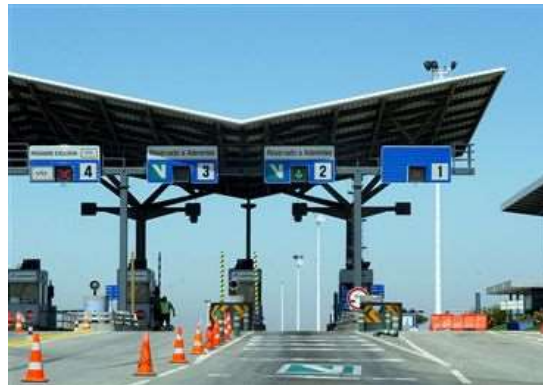
Example of VIA VERDE toll station
