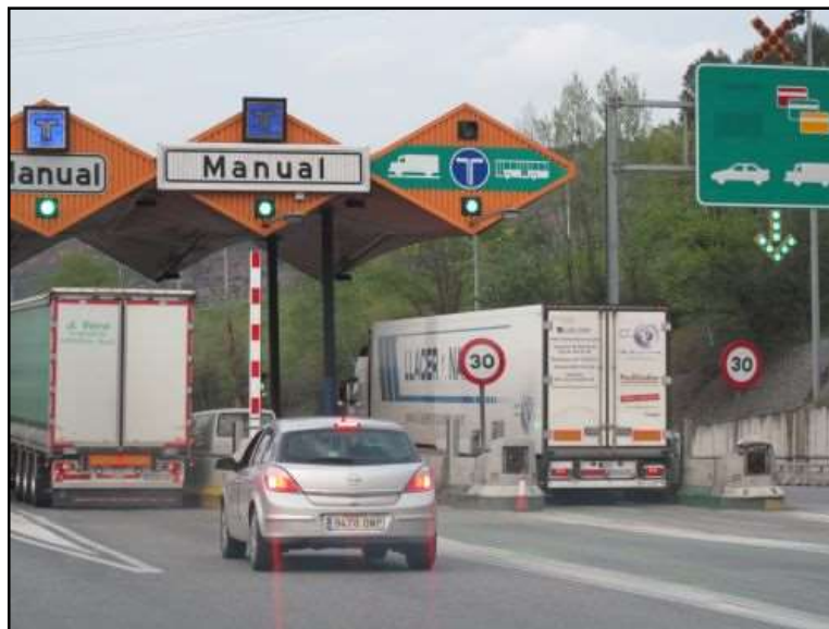
Example of a VIA-T station
